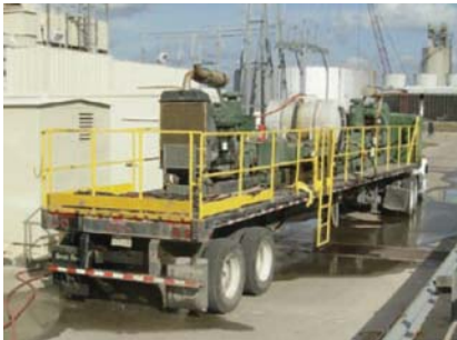
E. Hydrolazing is no small task; flatbed holds all equipment required
