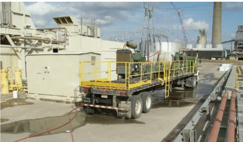
E. Hydrolazing is no small task; flatbed holds all equipment required
